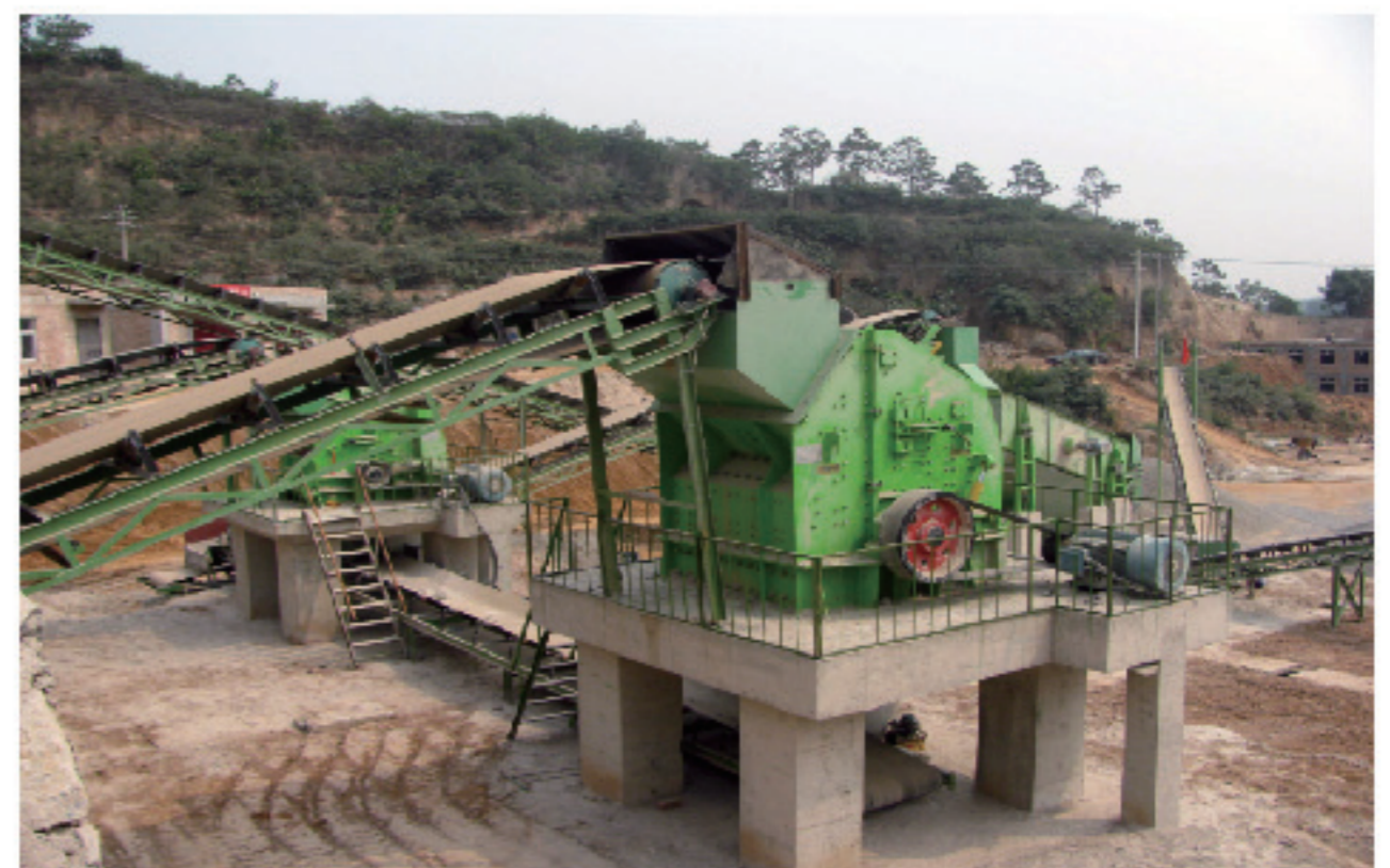
反击式破碎机在加工砂石骨料 Impact crusher is producing aggregates
